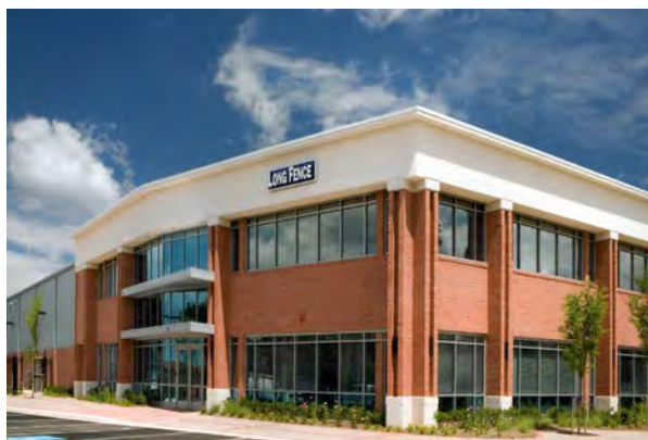
Long Fence Headquarters, Odenton, MD
